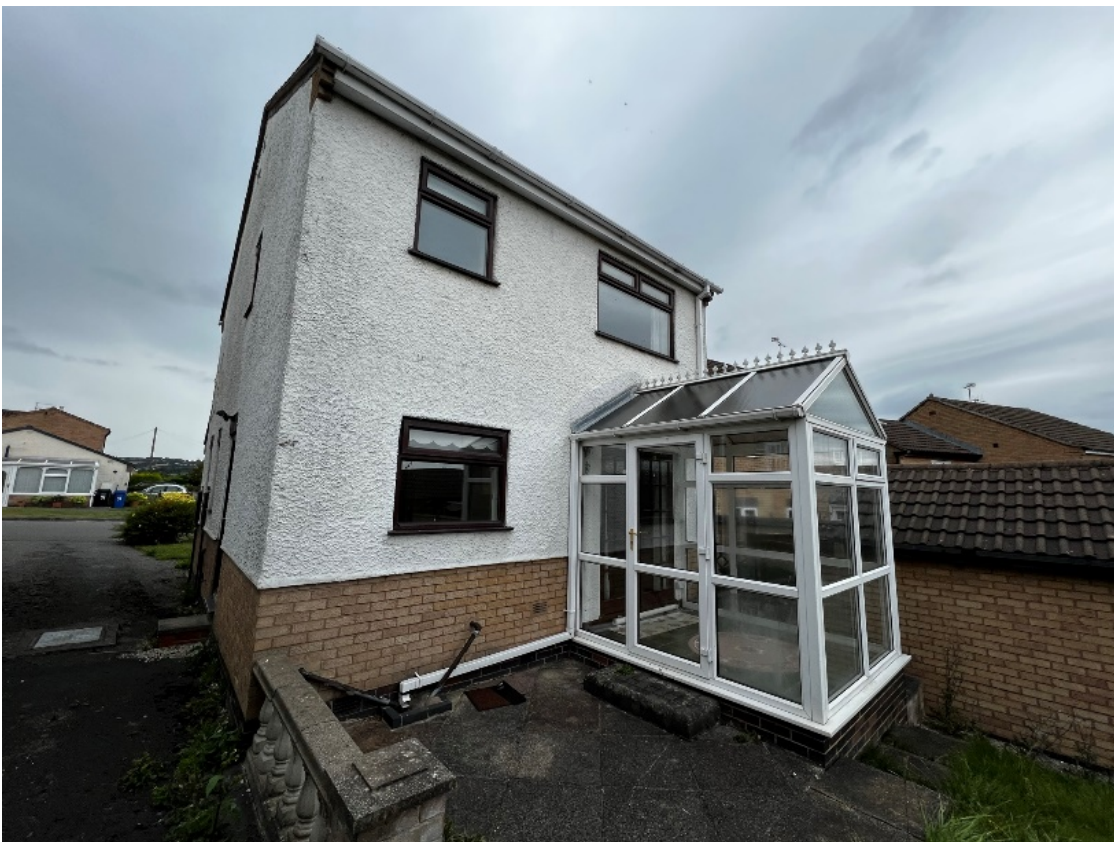
Figure 3 - showing the rear elevation of the site dwelling with the conservatory which would be removed
