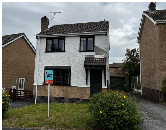
Figure 1 - showing the main front elevation
